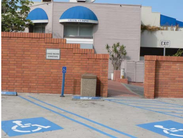
On-site parking connects to retail by a pedestrian-friendly alley in Laguna Beach.
